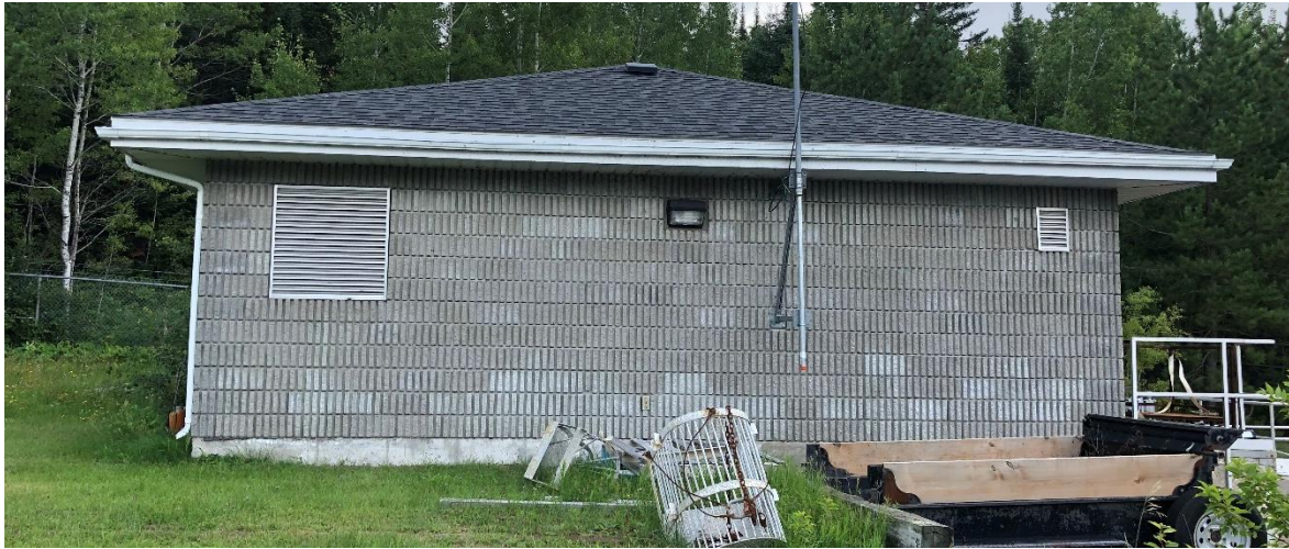
Facility – North-West Façade
