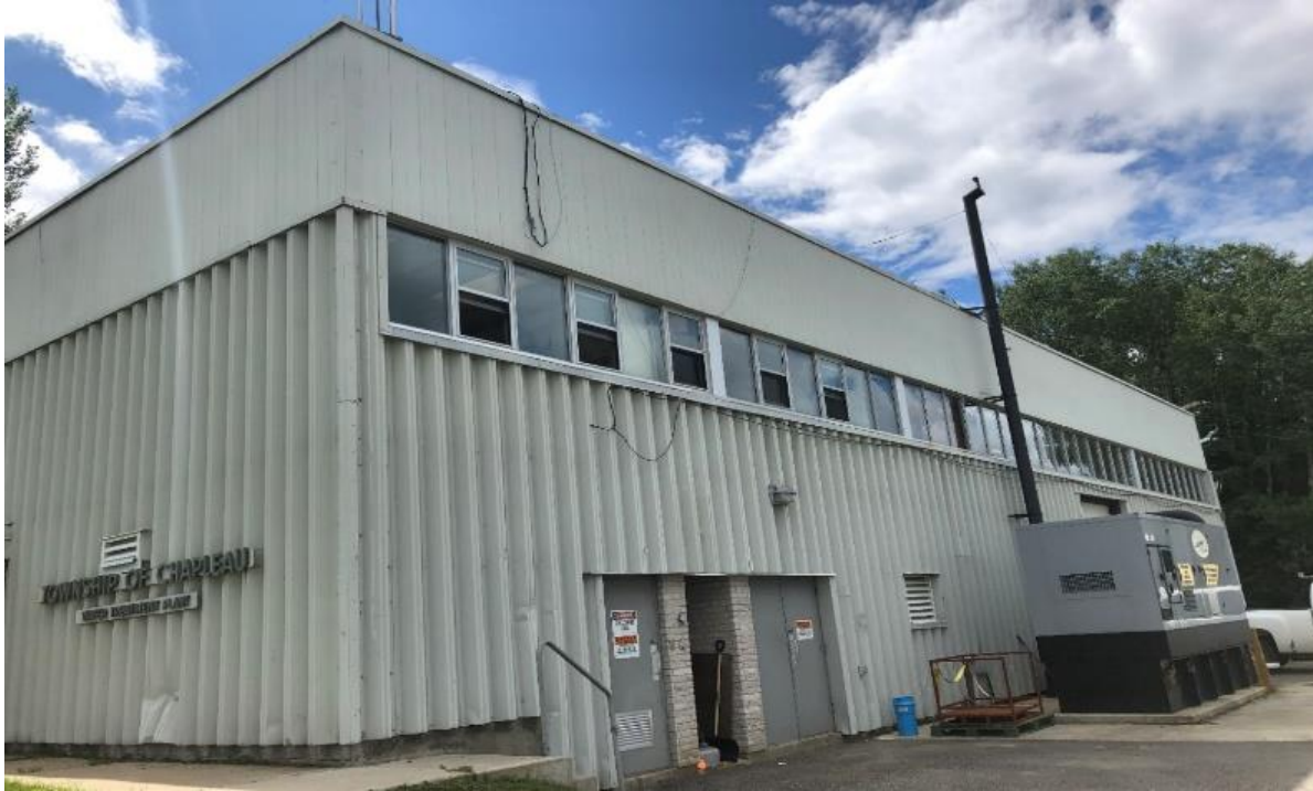
WTP - North East façade
