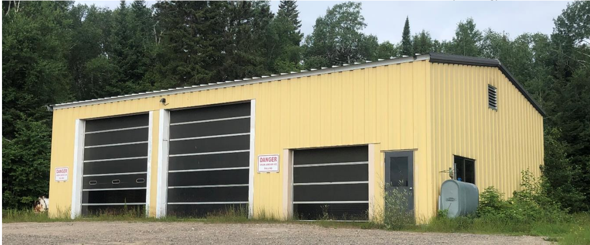
Garage – South East Façade
