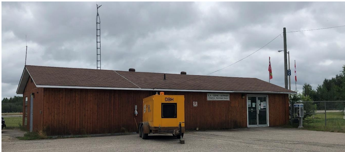
Terminal – North-West façade
