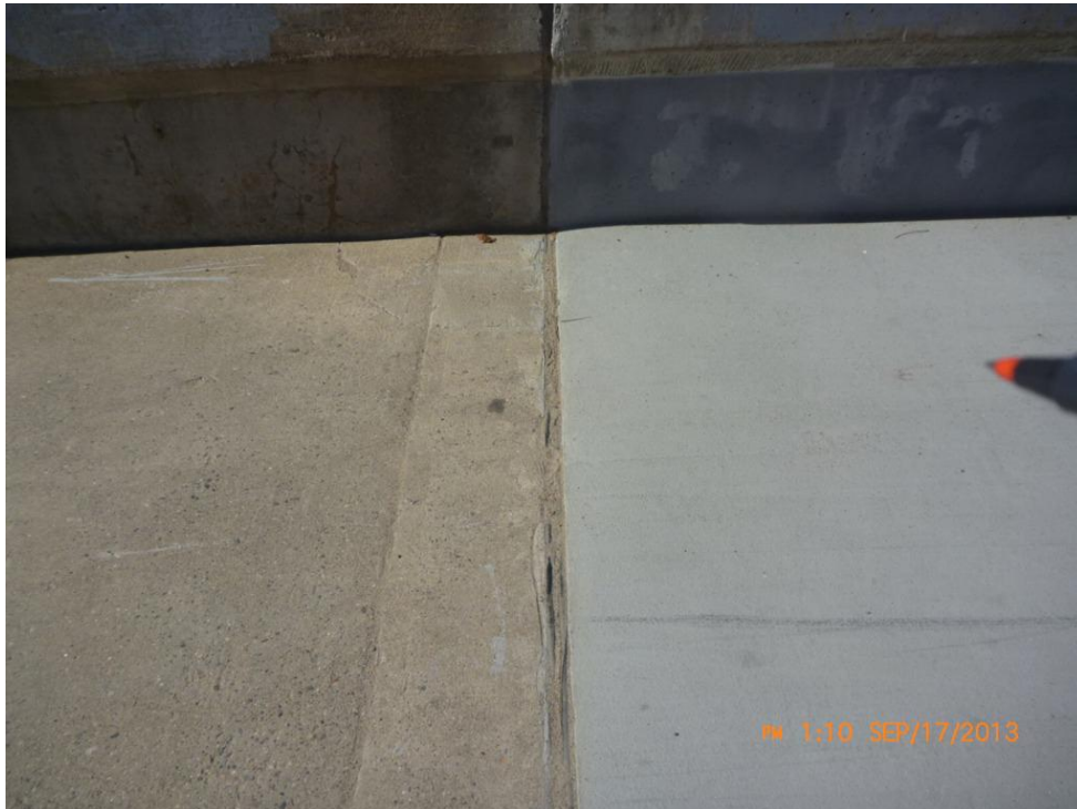
Comments: WEST EXPANSION JOINT
