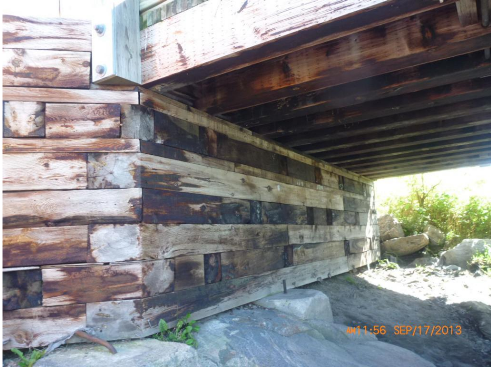
Comments: EAST ABUTMENT WALL
