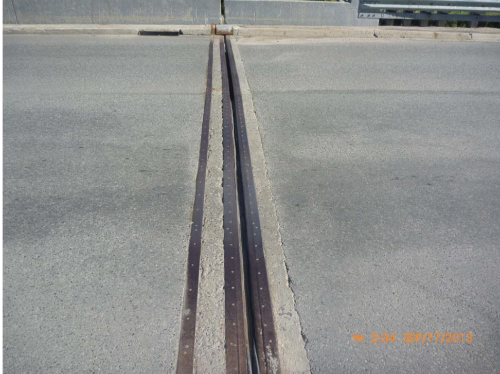
Comments: WEST EXPANSION JOINT
