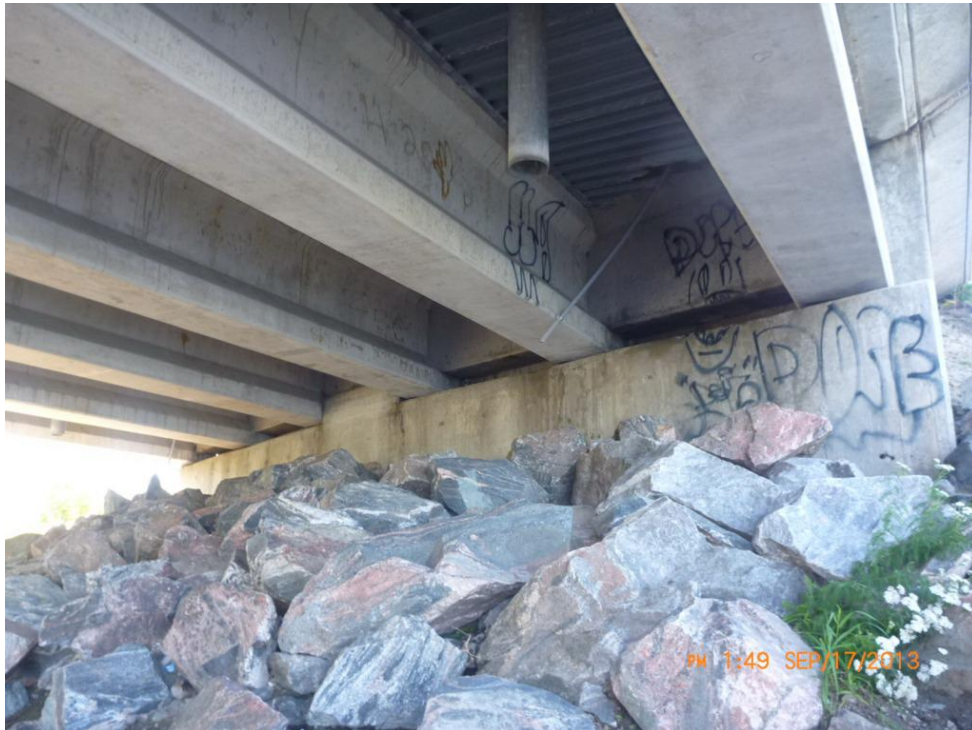
Comments: NORTH ABUTMENT
