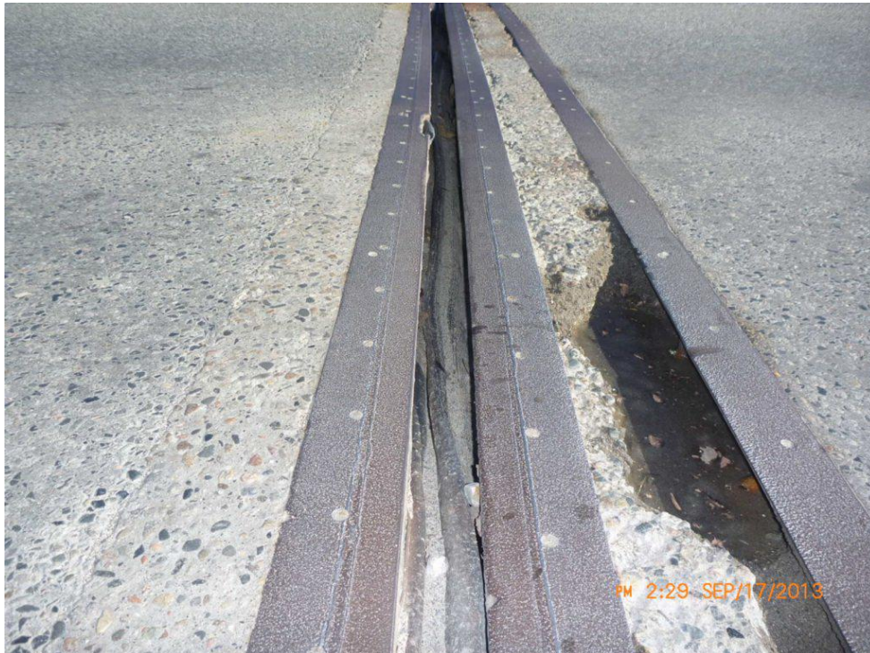
Comments: TWISTING OF EAST JOINT SEAL
