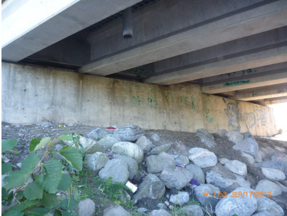
Comments: SOUTH ABUTMENT WALL
