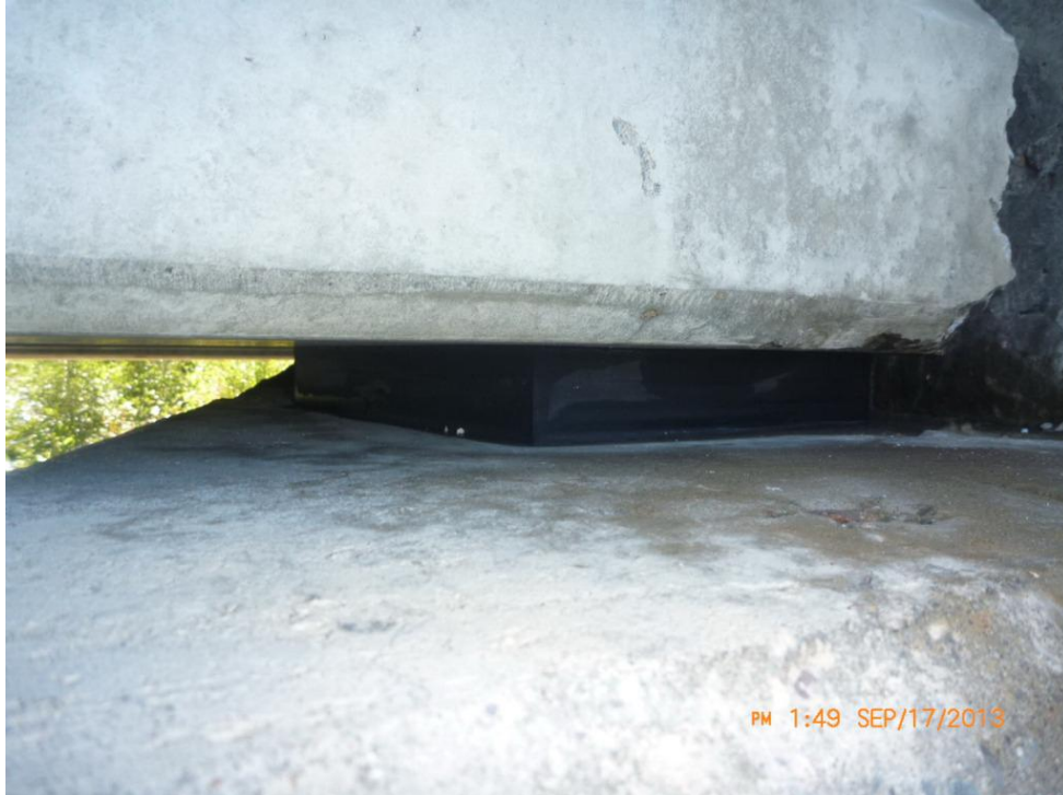
Comments: TYPICAL ABUTMENT BEARING
