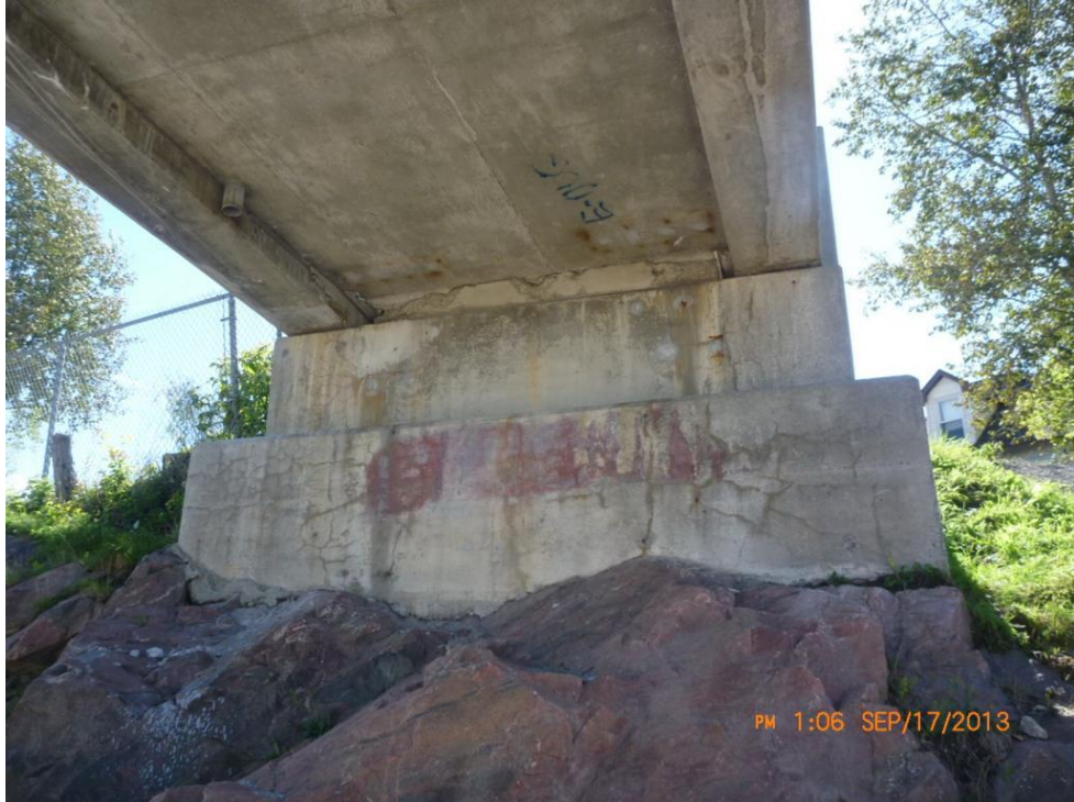
Comments: WEST ABUTMENT WALL
