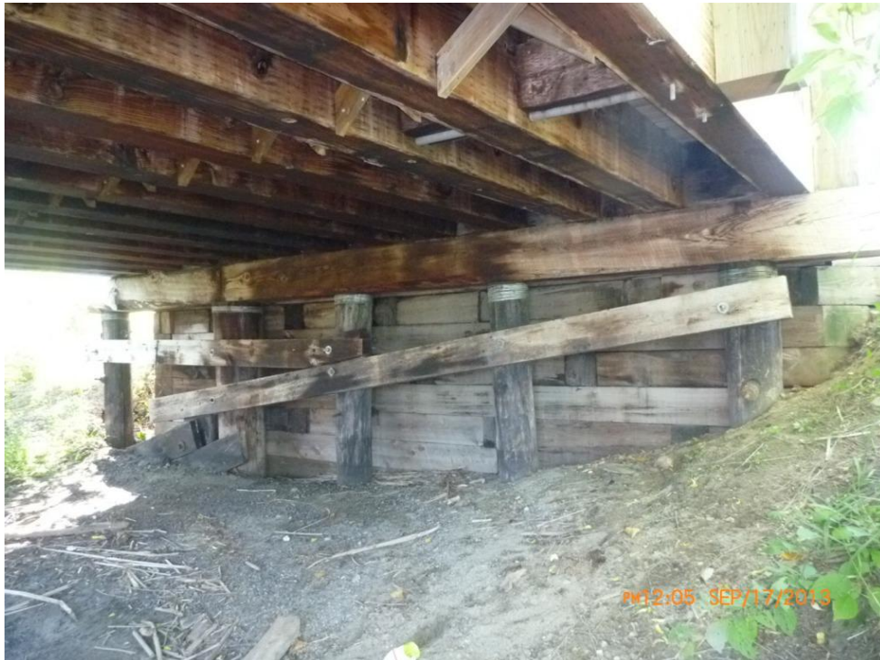
Comments: WEST ABUTMENT WALL Path: E:\WorkTech Data\Chapleau\Photos\2013\Photo 015.JPG
