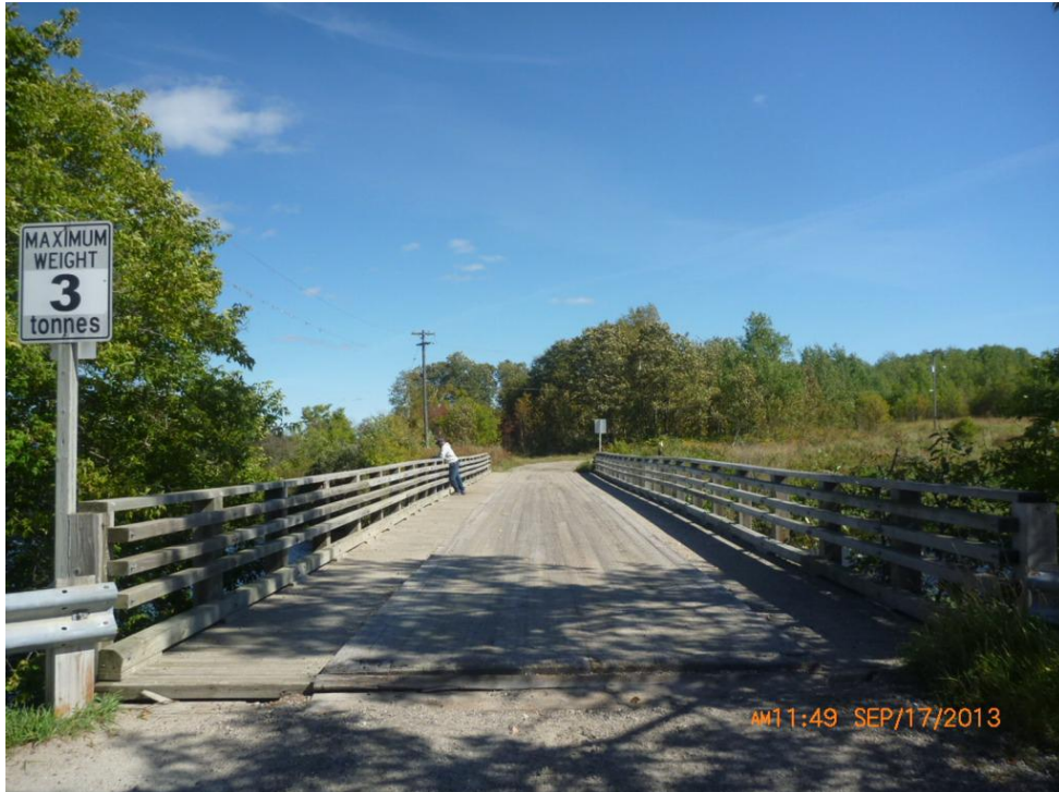
Comments: LOOKING EAST OVER STRUCTURE
