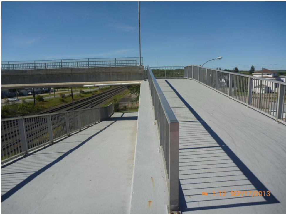
Comments: LOOKING NORTH AT PEDESTRIAN WALKWAY
