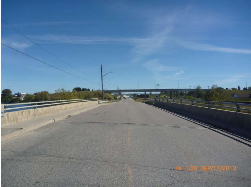
Comments: LOOKING SOUTH OVER STRUCTURE
